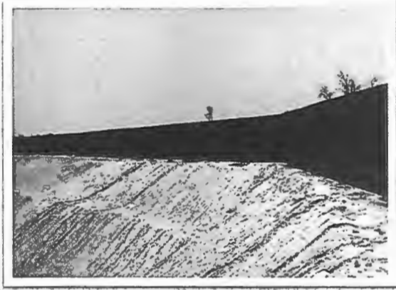
Wind breaking wall & profile sheeting around siding
