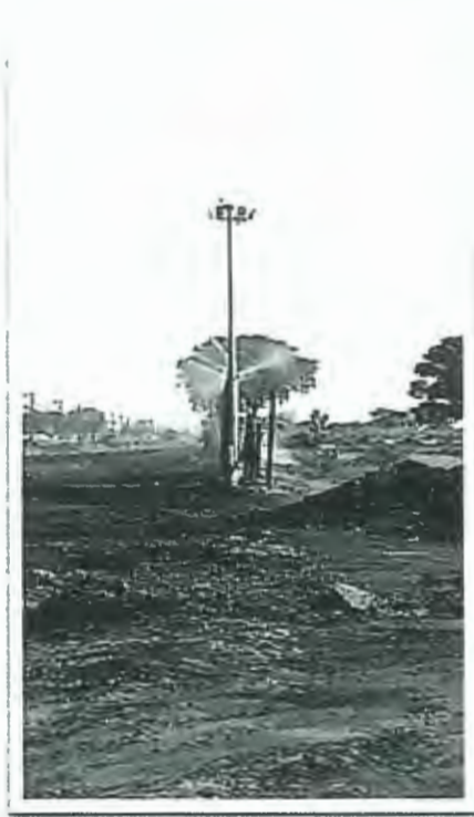
Water Sprinkling System at Bargawan
