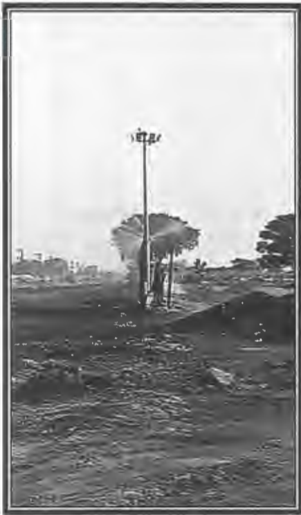
Water Sprinkling System at Bargawan
